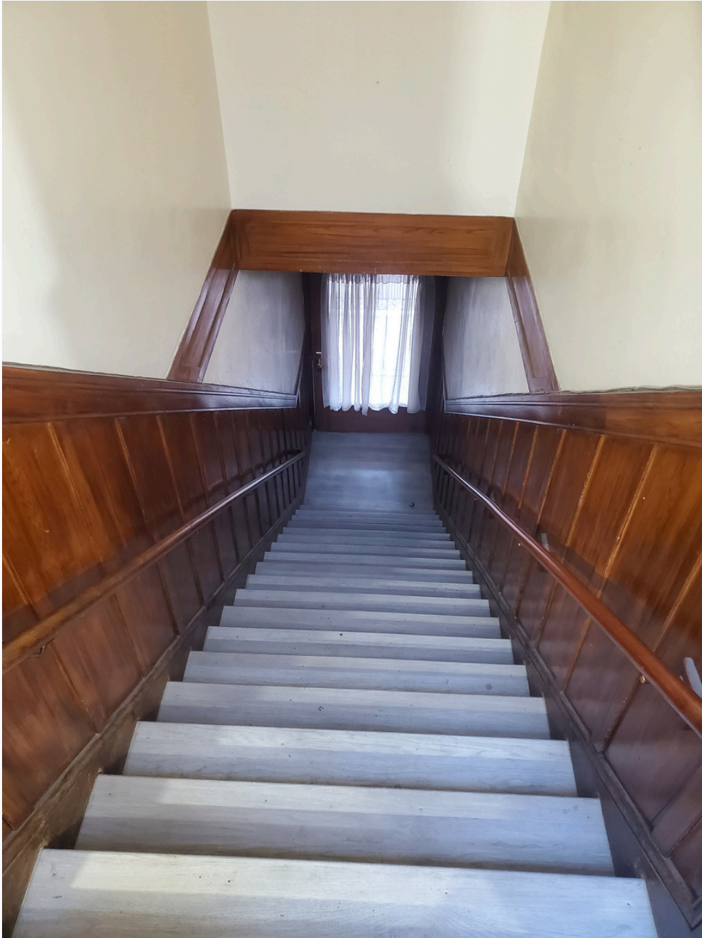
Stair to access the second floor
